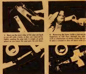
4. Quickly give the fitting a light but thorough coating of solvent full depth of the socket. This wash gunk in the fitting will block the passage but enough remains. Check after assembly.
